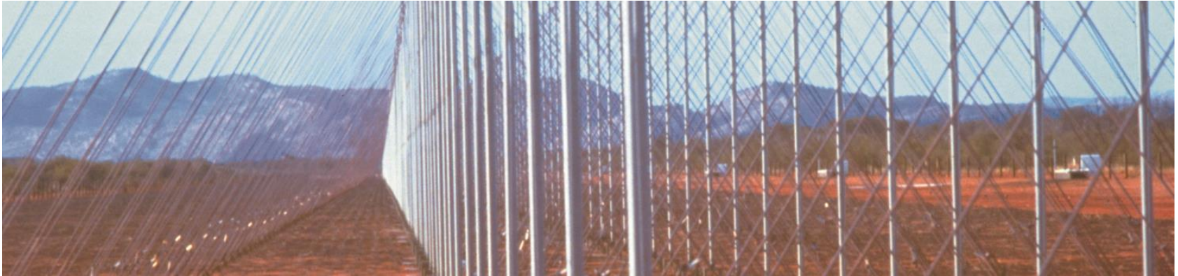
Jindalee Over-the-Horizon Radar
